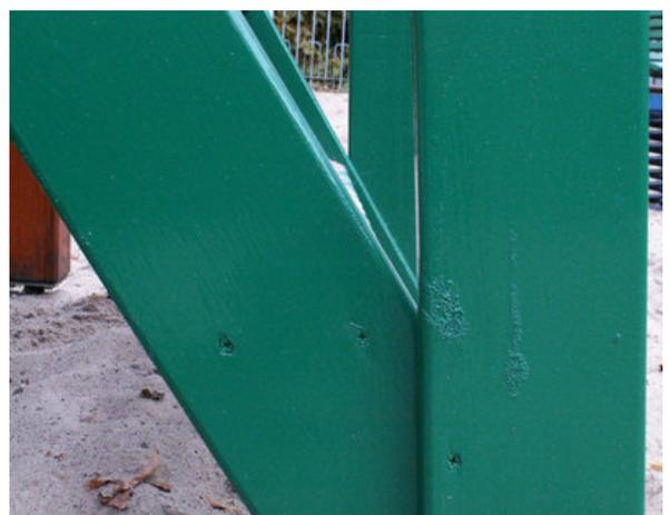
**7.13 Head and neck entrapment.** Head and neck jamming can be examined above 600 mm, and on carousels, for two types of openings: open and close type.
