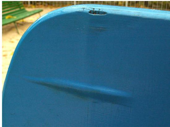
**7.10 Deformed or damaged elements.** During examination one should take into consideration the irregularities caused by wearing through, as well as unintentional or deliberate operations, e.g. cut ropes, damages to wooden elements which occurred during grass cutting and other operations, damages caused by animals or by usage of equipment which violates their destination. Please, write only those faults which have not been included in other sections!
